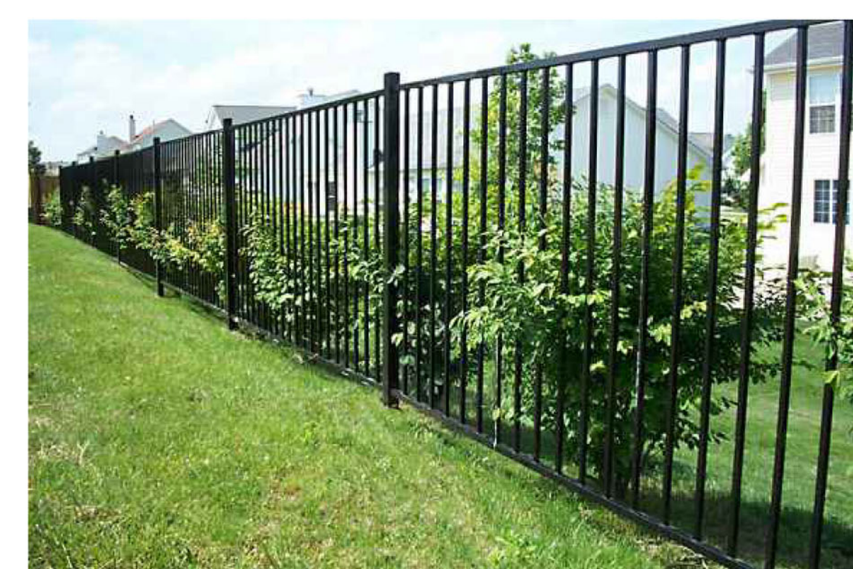
TUBULAR STEEL FENCE
